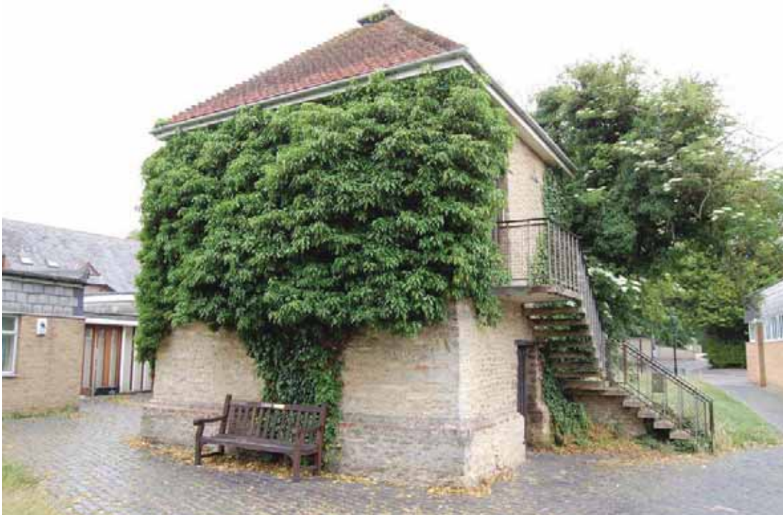
Plate 1. Existing priory structure, the dovecote.
