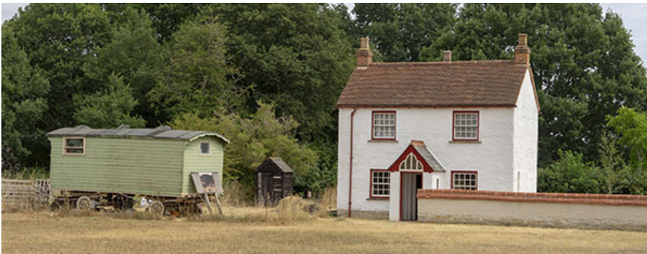
Haddenham Croft Cottage - Originally built in the 1830s. The walls are made of a special type of local earth called Wychert.
