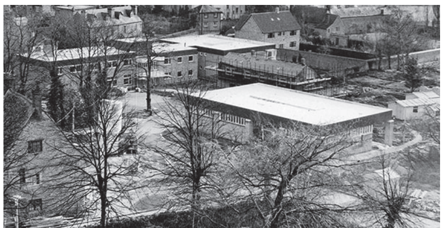
The current library in Old Place Yard, under construction. - 1965
