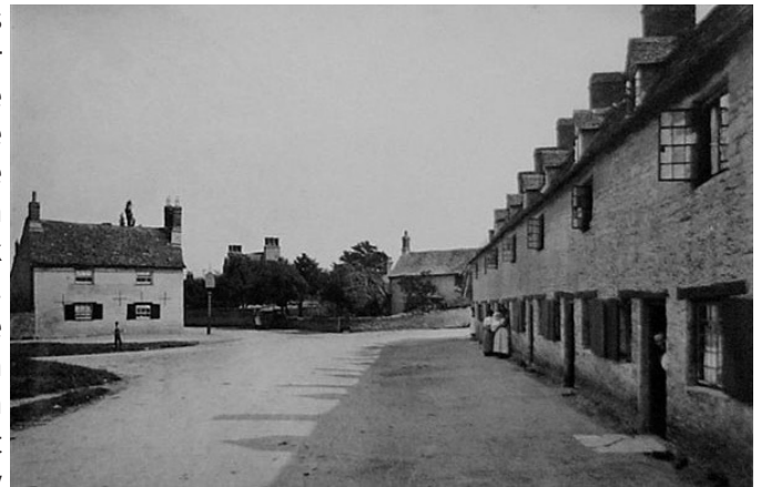
View looking south along the west side of the village green.
