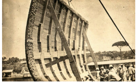
HMS Dartmouth's coffer dam being lifted into place.
