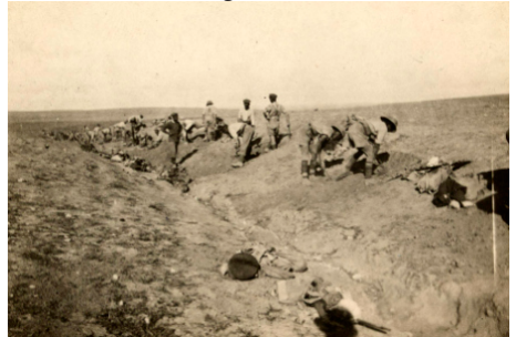
Trench digging in the Sinai Desert.
