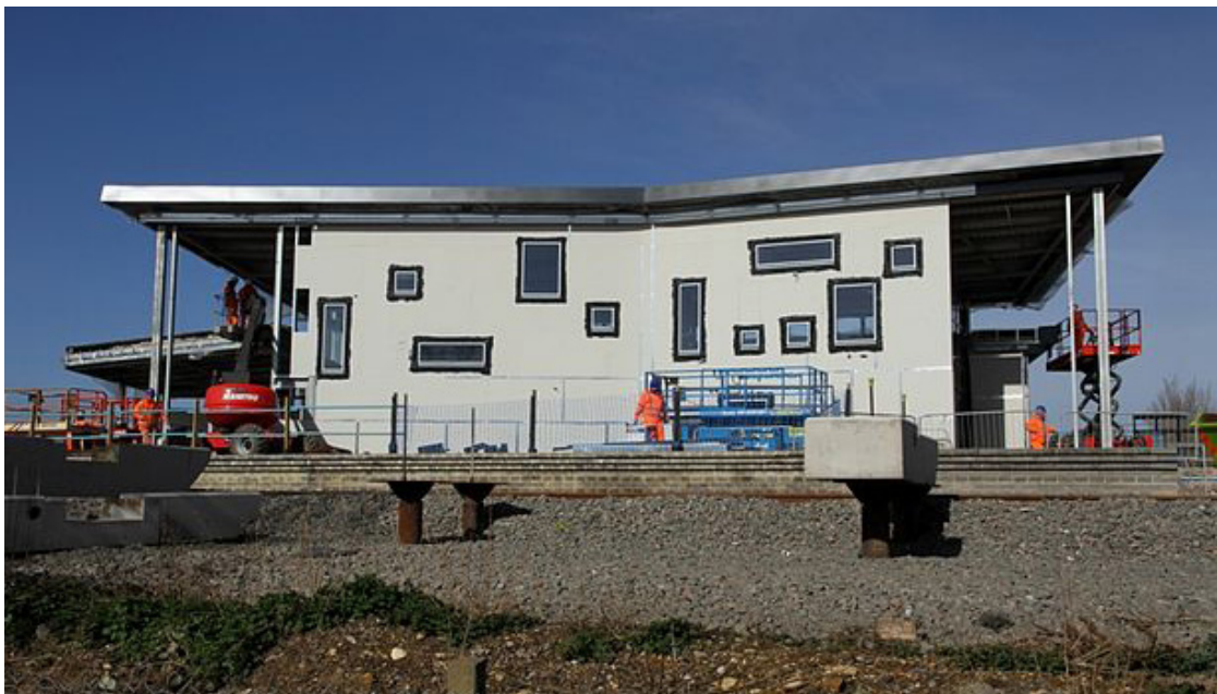
New station building under construction - 2015
