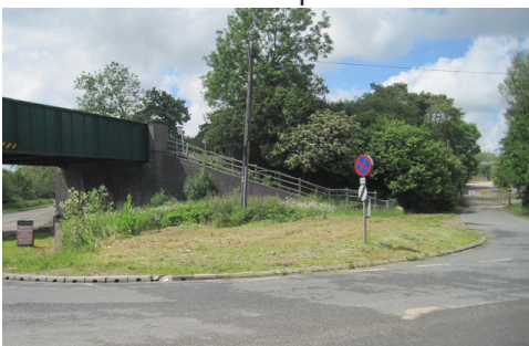
Site of Blackthorn station, just off the road to Marsh Gibbon.
